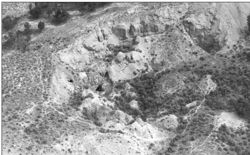
Large sinkhole (diameter approx. 200 feet) in Eagle Valley Evaporite near the Eagle County Airport outside of the town of Gypsum
