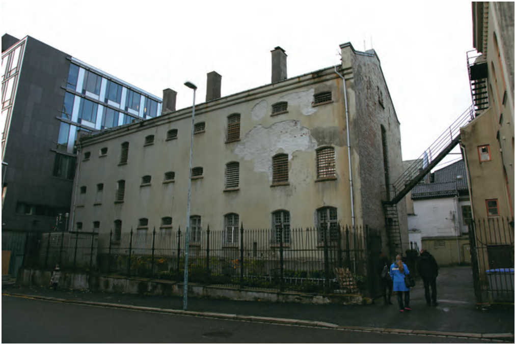
Old county jail, Bergen, Norway.
