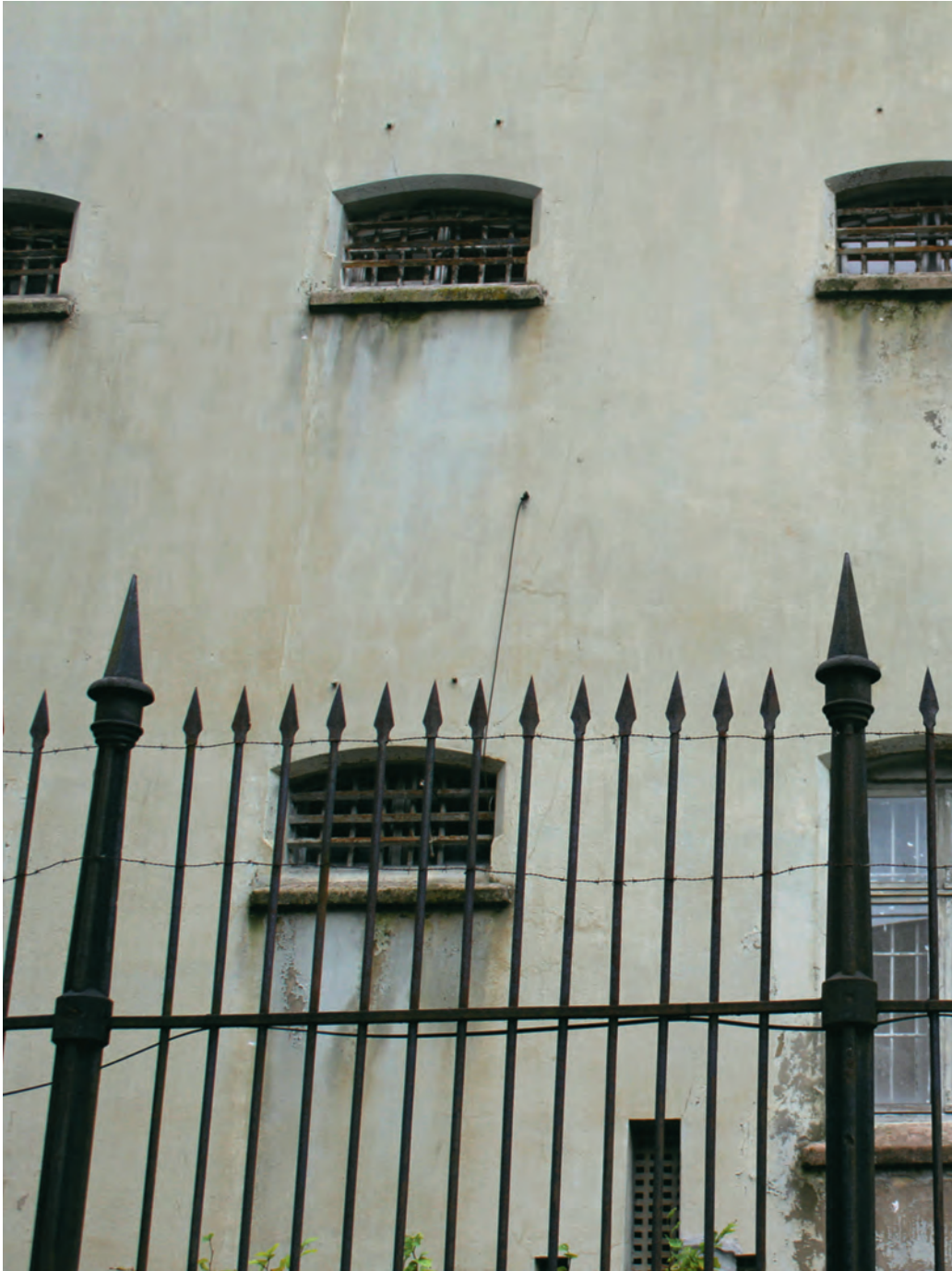
Old county jail, Bergen, Norway.
